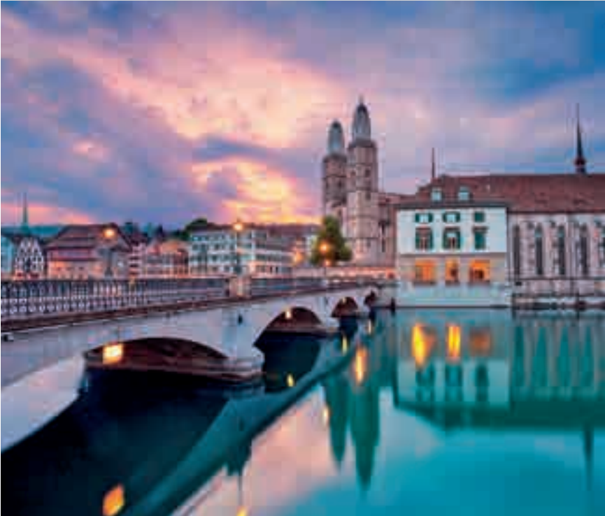
Munsterbrücke spanning the Limatt River
